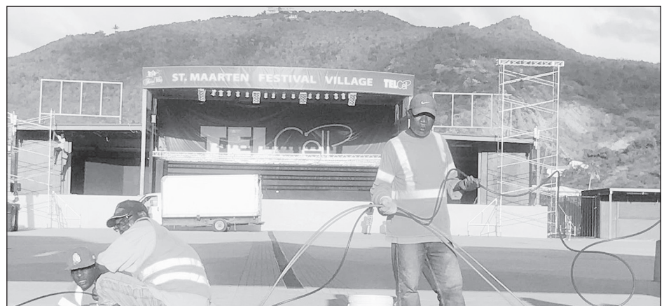
TelEm uses local contractors to pull fiber-optic cables to the Festival Village and surrounding areas. Photo contributed
